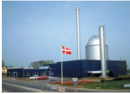
Power Plants, Diesel/gas engine (built by Wärtsilä)
